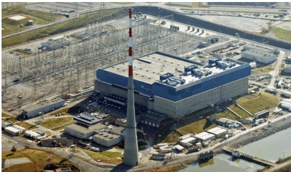
Browns Ferry Nuclear Power Plant, USA
