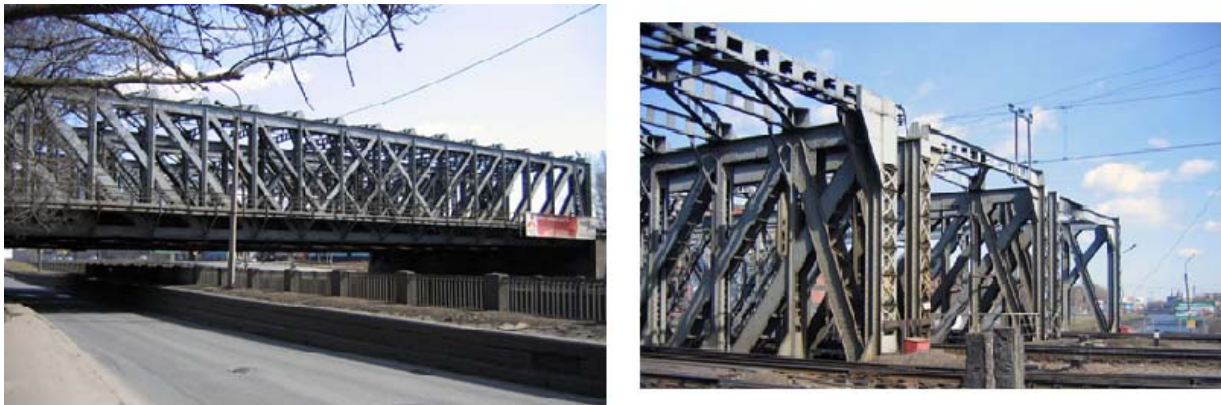
Image 1 – American bridges before reconstruction
