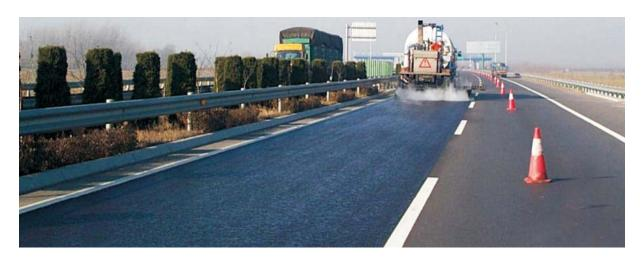
2. Rejuvenator Seal is a technology which is similar to Fog Seal. The difference is that instead of emulsified bitumen for impregnation of asphalt covering special rejuvenate composite is used. Such kind of impregnation protects covering from deterioration and renovates its surface. Rejuvenator Sealing is also used in asphalt covering, which have axial and transversal fractions and provides inactive crack healing. This technology prolongs covering life cycle for 1-3 years till overhaul.
