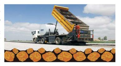
Upgrading with the use of hot bitumen as binding is explained by the fact that for so short period of time bitumen does not have time to cool and preserves thin consistency and high adhesive capacity. As a result bitumen is well pierced to breakstone and covering micropores, obducing each chip and firmly pastes them to covering and one to another.
