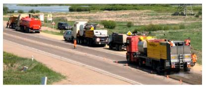
Cape Seals can be used as a protecting layer of the covering which is arranged on a long term for a heavy traffic covering and also for cracks elimination.
