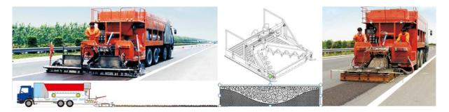
Macro-Surfacing is one of the technology variation. It is a porous cold composite, which consists of one breakstone fraction, plastic modified binder (emulsified bitumen), fine aggregate and special additives. This composite is similar to Slurry Seal, but is applied in specific cases, where it is important to provide noise reduction, good drainability and to reduce the probability of reflected cracks occurrence. This technology prolongs covering life cycle for 2,5-6 years till overhaul.
