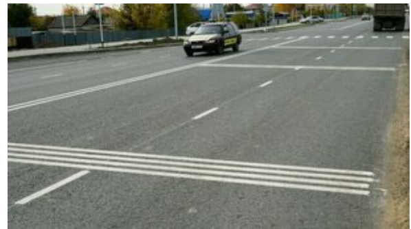
Figure 8 – Installation of noise strips before a pedestrian crossing [6]
