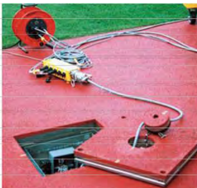
Extraction of cable from hand hole (2)
