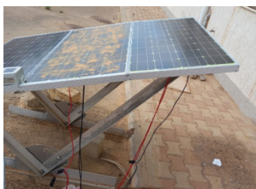
Figure 3. Installing the solar panels
