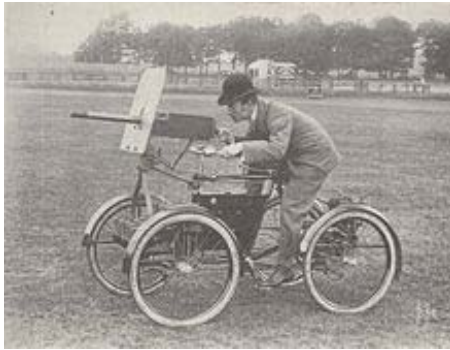
Fig. 15.1. F. R. Simms' Motor Scout, built in 1898 as an armed car
