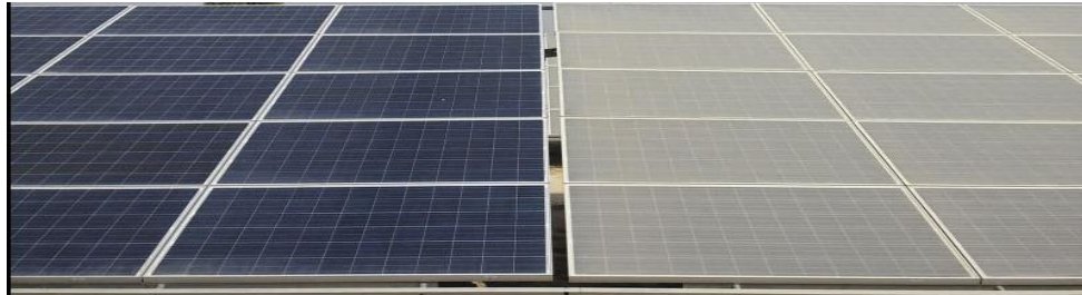
Figure 1 – Impact of dust on solar panels
