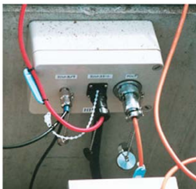
Connector box installed in hand hole (2)
