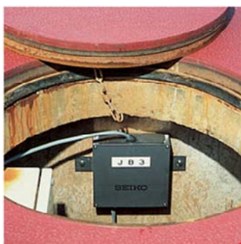
Junction box installed in hand hole
