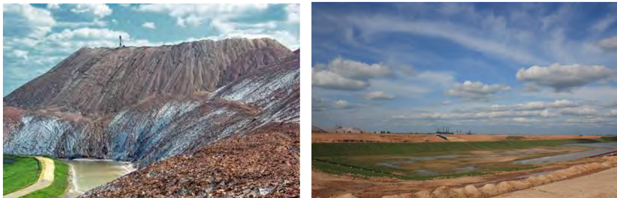
Picture 1 – Technology-related zone in the vicinity of salt dams (a) and sludge storage tanks (b)
