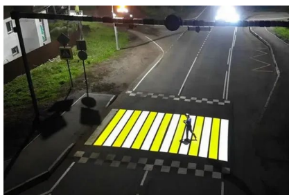
Figure 9 – Projection road markings on pedestrian crossings [8]
