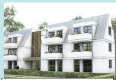
Residential Building in Nemencine Highway Vilnius, 2017
