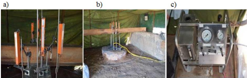
Figure 6 – Testing of piles by static load using the O-cell method: a – fixing the displacement sensors; b – an experimental pile and a reference system c – hydraulic system (O-cell jack) [12-14]
