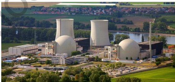
Biblis Nuclear Power Plant, Germany
