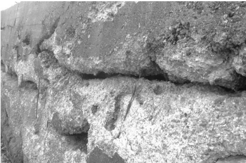
Fig. 3 The front wall of Kholmsk port berth facilities
